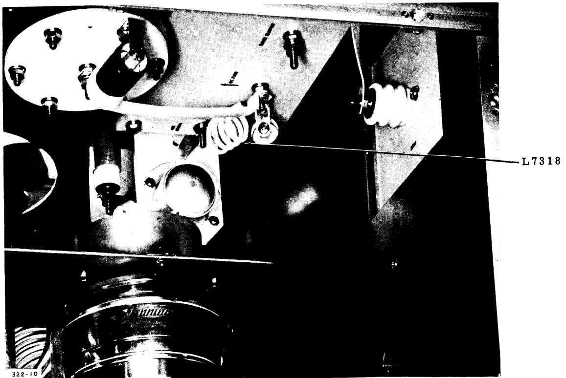
Figure 3-2. Connections for 10-kw Emergency Operation
