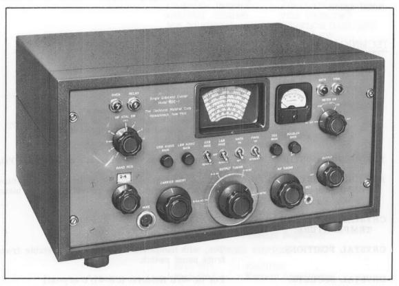
The TMC Model SBE-1, Mode Selector, Transmitting, is a universal exciter permitting the transmission of any intelligence on Single or Double Sideband, with or without carrier.
